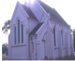
h00599 st marks anglican church albert st rosedale south eastern profile she project 2003
