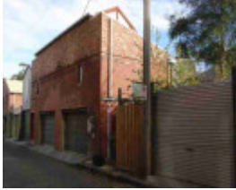
fitzroy little smith street fitzroy little smith street 143
