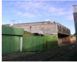
Rear of 91 Clauscen Street.JPG
