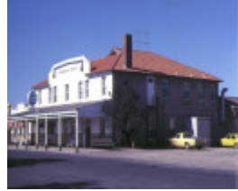
1 rosedale hotel lyons street rosedale rear view of hotel feb1982
