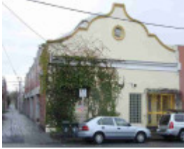
fitzroy westgarth street fitzroy westgarth street 93 unit 2
