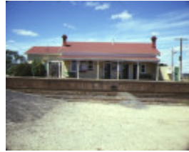
1 rosedale railway station complex willung road rosedale front view feb1985
