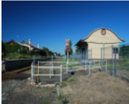
ROSEDALE RAILWAY STATION COMPLEX SOHE 2008
