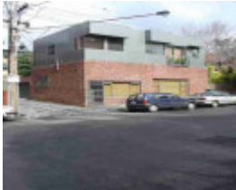
fitzroy hanover street fitzroy hanover street 14
